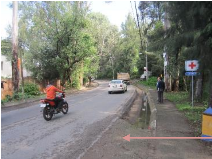
Km 36+320 (toma norte a sur)
